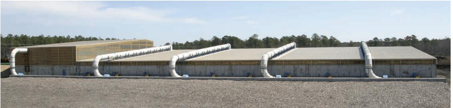
McGill-Sussex plant is the largest enclosed composting facility in Virginia. Biofilter (foreground) removes odors and particulates from plant exhaust.
